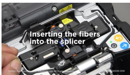
Inserting the fibers into the splicer
