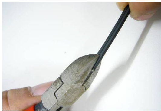
4: Make a slit along the groove of the cable sheath using nippers.
