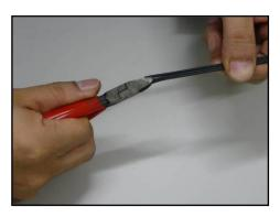
1: Separate the steel wire from the cable using nippers.
