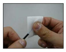
3: Clean the bare fiber from the end of the fiber coating with a gauze pad moistened with pure alcohol. Pull the bare fiber through the gauze pad and rotate the fiber to remove any coating residue.
