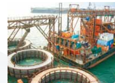
Off-loading power cable for transshipment for Lamma Project
