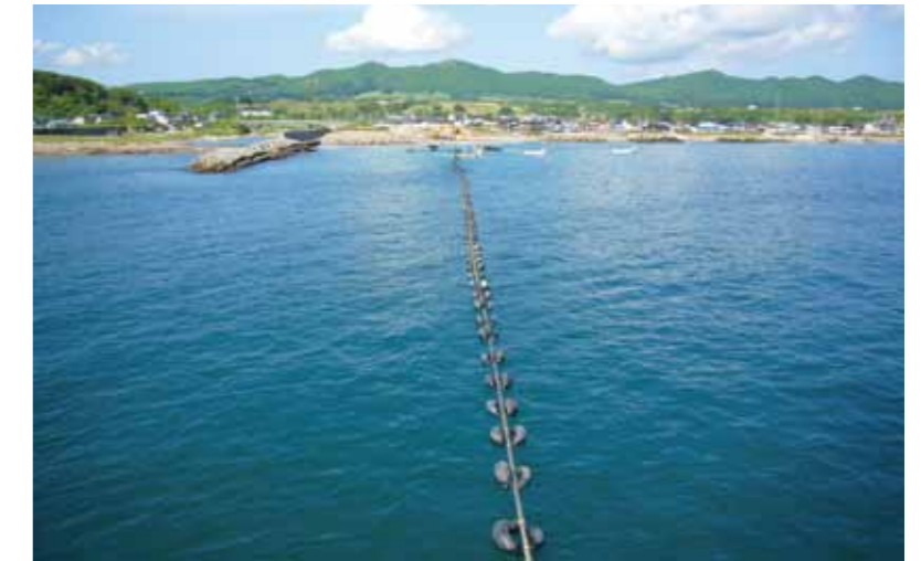
Cable installation of DC250kV XLPE cable in Hokkaido
