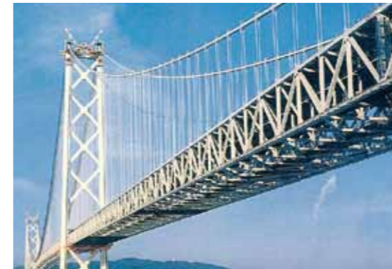
77kV XLPE cable installed on the world's longest bridge in 1998
