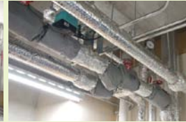
Thermal insulation of steam pipes
